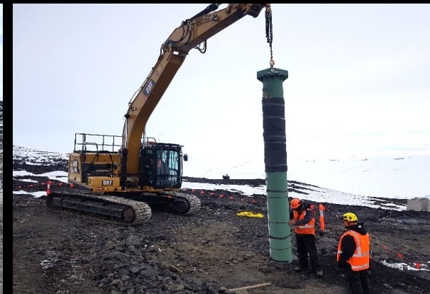
Pile trial on site
